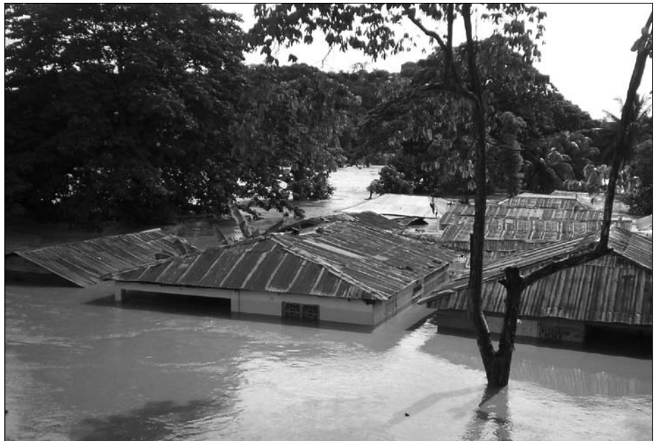
Flooding destroyed entire communities in Hinche.
